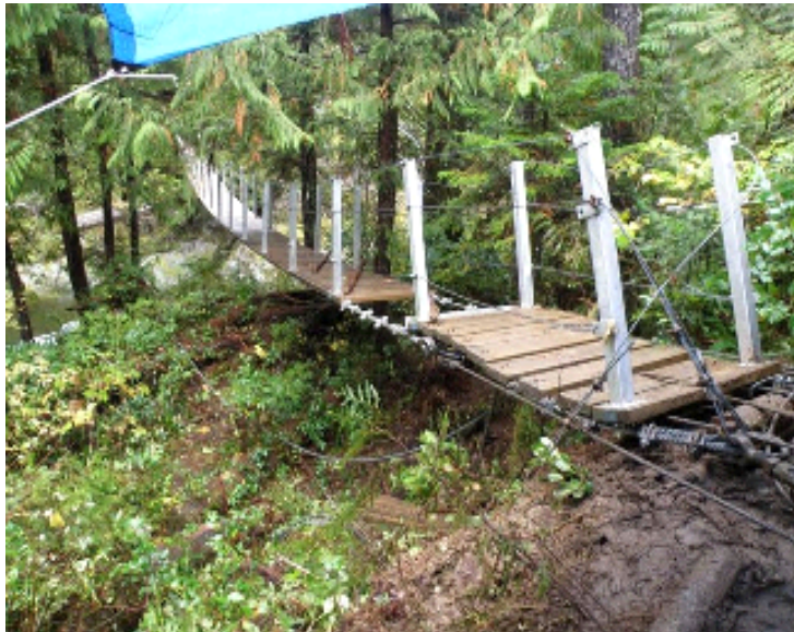
Bridge repairs almost complete
